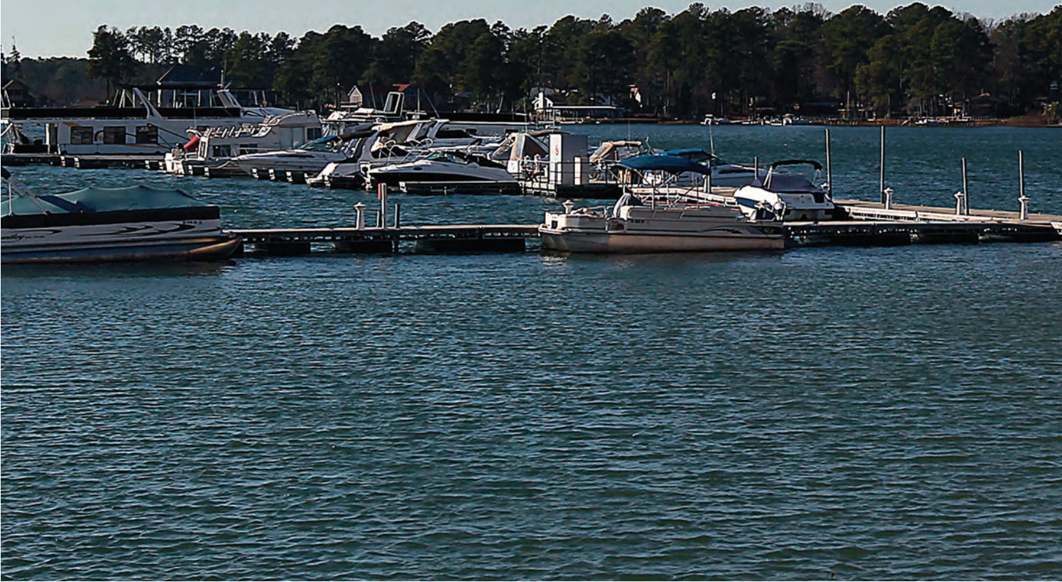
Life and leisure. Liberty on the Lake, a waterfront bar and grill is under construction. Inset, what the complex should look like upon completion.
